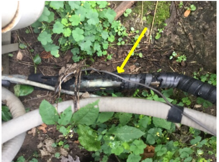
Insulation is deteriorated or missing on the suction line at exterior of house, recommend replacement of insulation to maximize the efficiency of the unit.
