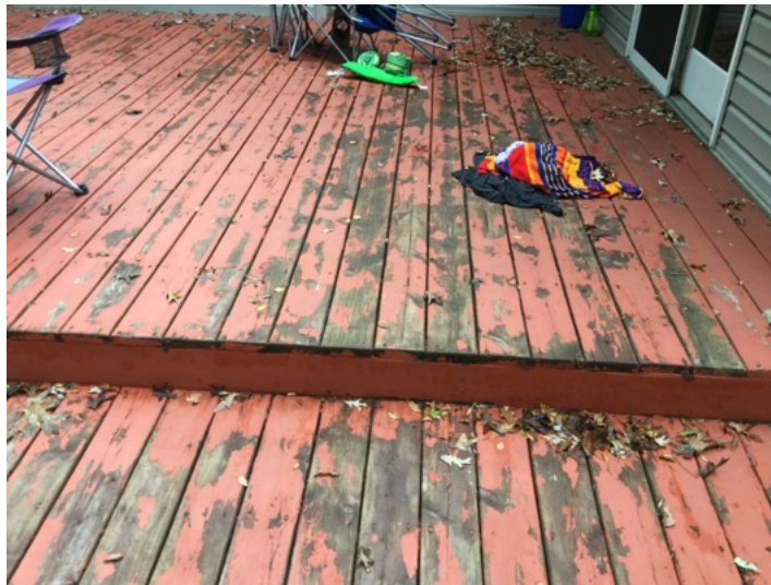
clean and seal the deck.
